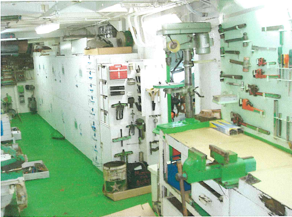
Engine room workshop
