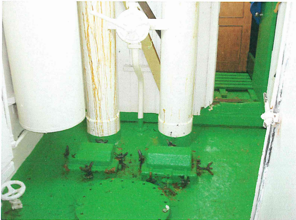
Forward chain lockers and accommodation
