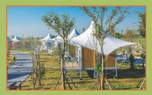
Container Size: L5800xW4600xH2500mm Tent size: L7400xW8400xH4800mm Outside balcony size: 5800\*2000mm Structure : steel structure + fiberglass sandwich panel + insulation + decorations Configurations : balcony deck , steel supporters , roof tent , water heater , bathroom fully fixtures, electrical and water plumbing Transport: 1\*40ft HQ\_load 1 unit
