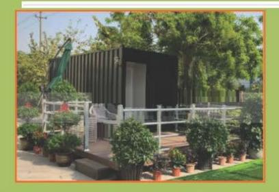
Size: L6058 x W2438 x H2591mm Structure : modified ISO 20ft shipping container, sandwich panel decoration and insulation Configurations :Bathroom fully fixtures, wardrobe, bed, computer desk and chair, electrical and water plumbing system Transport : Shipped as ISO 20ft GP shipping container
