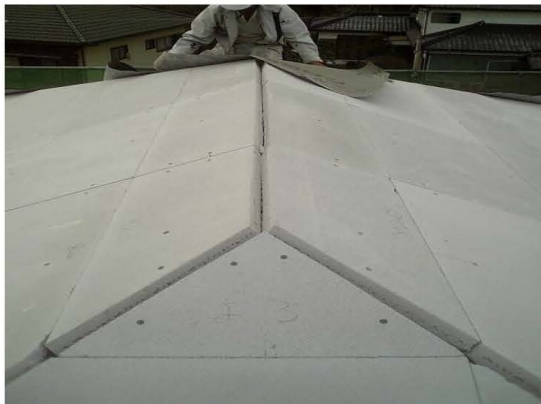
Roof wall panel
