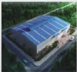
20000m 2 MARSHALL PLANT
