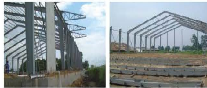
3500m 2 CONGO PROJECT
