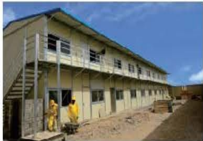
Dubai dormitory project
