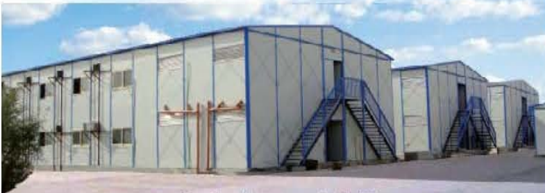
Dormitory labor camp project in UAE
