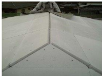
Roof wall panel
