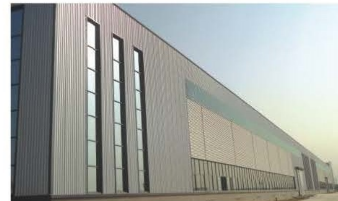
It has Lattice Column without anchor bolt which means a strict requirement for the steel column's perpendicularity, elevation and axis deviation. Column bracing has adopted welded channel steel and angle steel. The type of wall panel is V-780.
