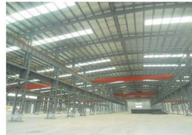
Leiting Heavy Industry Project The project of Leiting Heavy Industry is a structural steel warehouse, which is used as an assembly base for automatic transmission equipment for metallurgy industry. It is located in Qingdao High-tech zone, with length of 198.1m, span of 120m, eave height of 13.2m, and ridge height of 18.6m.
