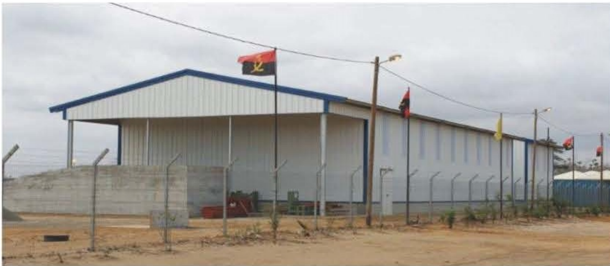
Cassava Factory, with the specification of 50m*15m*6m(L*W*H), mainly used for potato starch processing, which was built in Angola and completed in May of 2013.
