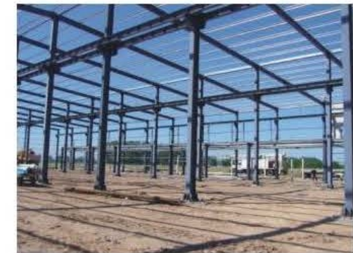
Light Steel Structure Workshop in Argentina Area: 5930m 2 Main Workshop: 80m*60m*9m(L*W*Eave Height) Affiliated Workshop: 1130m 2 Roof and Wall: V-960 steel sandwich panel Thermal Insulation: 50mm EPS Foam Density: 12kg/m 3 Wind Load: 0.79KN/m 2 Crane: 8 sets (Lifting Capacity: 2 Tons) Windows and Doors: E-folling Window & Door Project Site: Canuelas, Buenos Aires, Argentina Year of Construction: 2009
