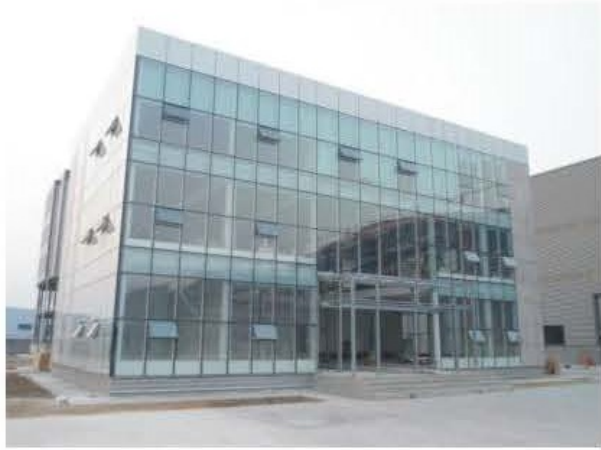
Comprehensive office building four layers, with the steel frame and glass curtain wall.
