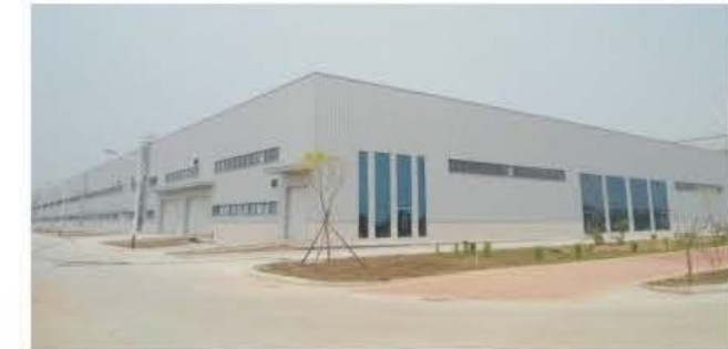
Leiting Heavy Industry Project The project of Leiting Heavy Industry is a structural steel warehouse, which is used as an assembly base for automatic transmission equipment for metallurgy industry. It is located in Qingdao High-tech zone, with length of 198.1m, span of 120m, eave height of 13.2m, and ridge height of 18.6m.
