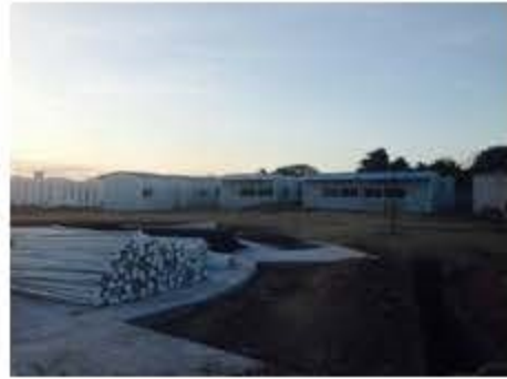
100 Units of Emergency Shelters after Cyclone Haiyan
