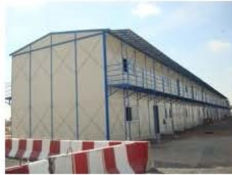
Dubai Fireproof Panel Worker Camp
