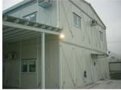
Hongkong K Modular Office
