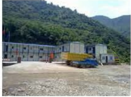
China Railway Construction Site Camp
