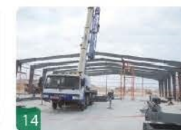
Steel structure installation
