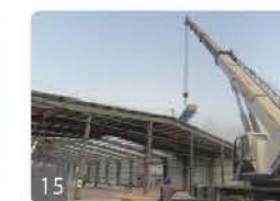
Roof and wall installation
