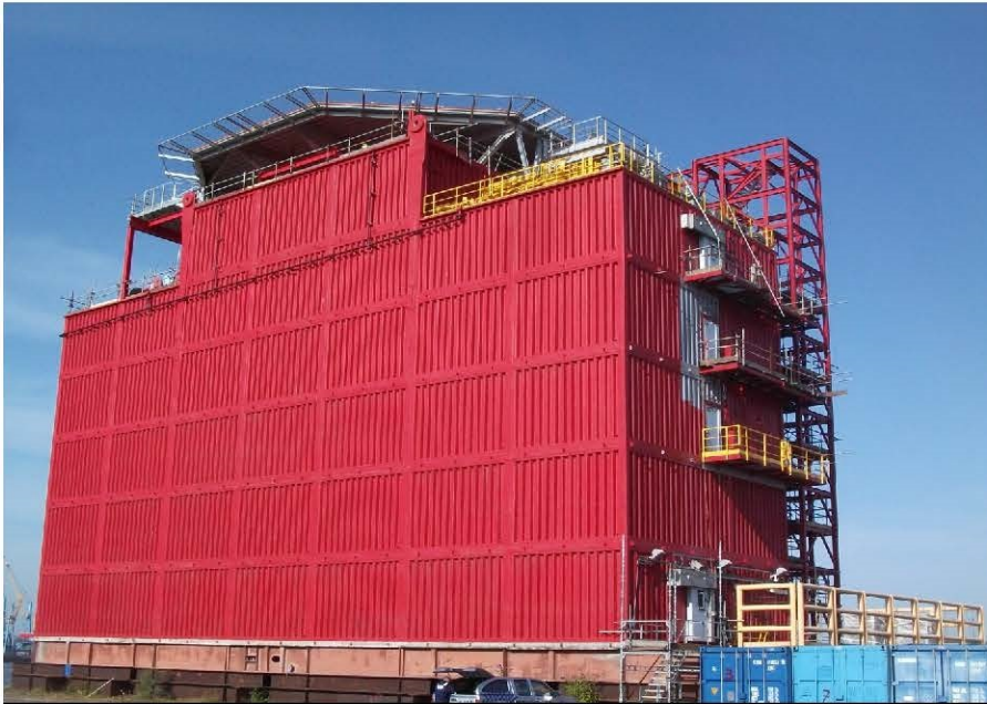
Exterior Back Overview of the 120 POB Living Quarters
