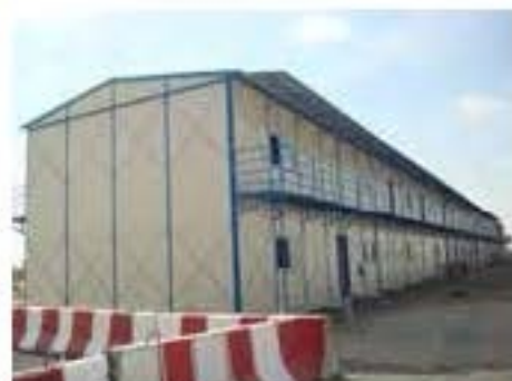
Dubai Fireproof Panel Worker Camp
