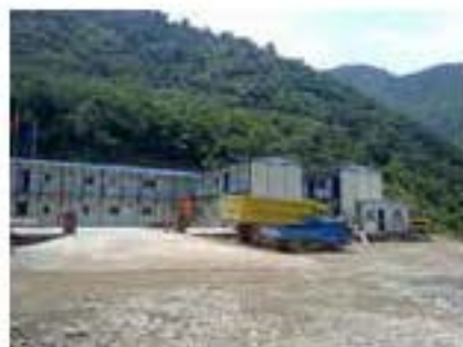
China Railway Construction Site Camp
