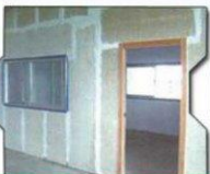
11. Installation of Door frame
