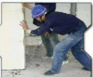
5. Positioning the panels
