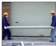
1. Carrying the panels
