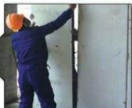
4. Panel erecting
