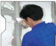
8. Installing crackresistant material
