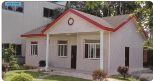
Light Steel Villa House
