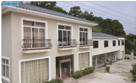
Light Steel Villa House
