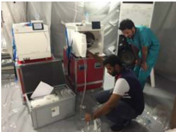
The sterilizers (left) and a double sink (right) in the CSSD.
