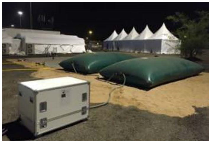
Filled clean water bladders are connected to a pump
