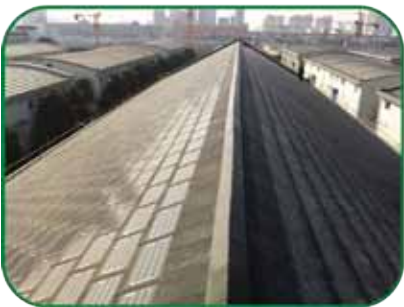
Install the counter batten and roof batten
