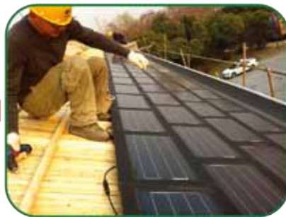
The photovoltaic tile roof is completed
