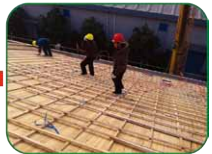
Cover the photovoltaic tile
