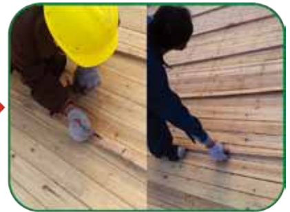
Do a horizontal line and test to check for level materials
