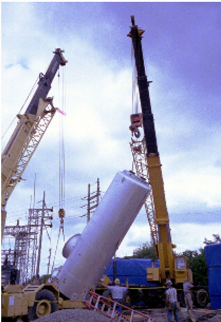
Positioning Lower Portion (noise muffler) of Exhaust Stack.
