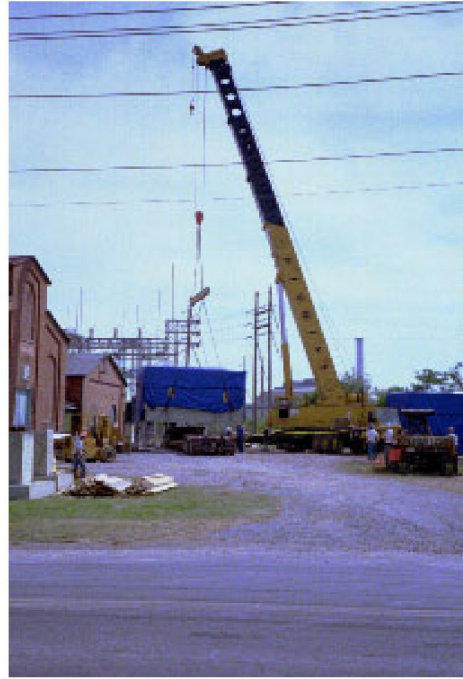
Lifting CT Unit from Flat Bed Trailer.
