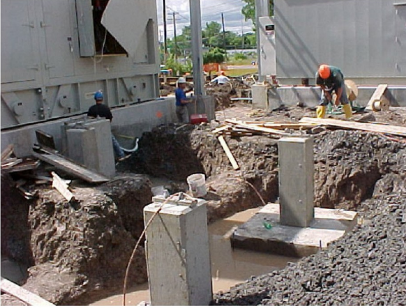
Foundation Columns for CT Air Inlet Structure.
