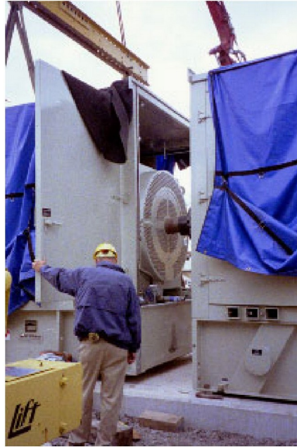
Setting and Aligning the Turbine and Generator.
