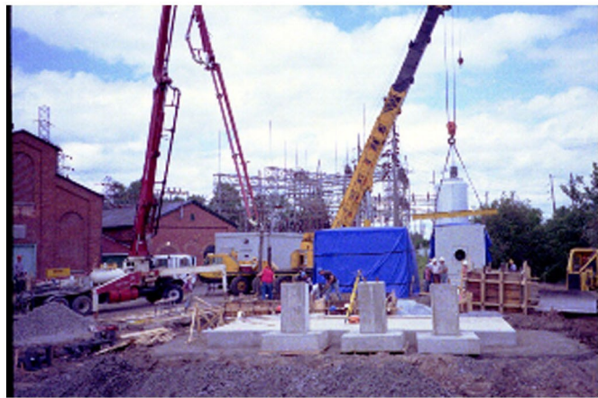
Setting the CT on Concrete Pad.
