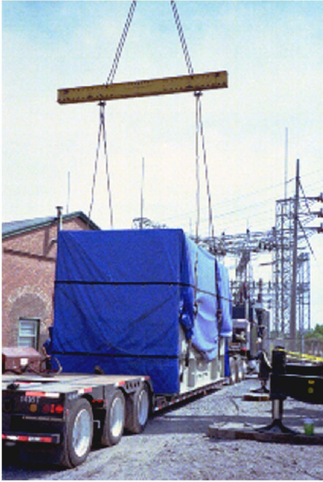
Arrival of CT at Auburn Site.
