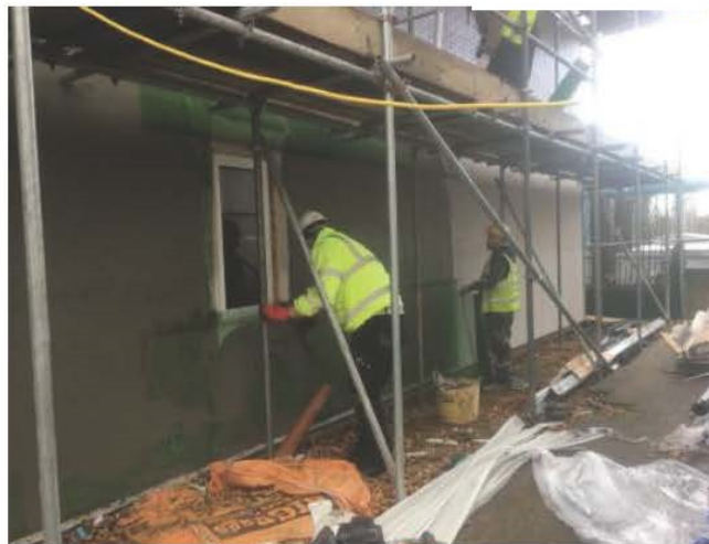
High density cement fiberboard and waterproof coating :
