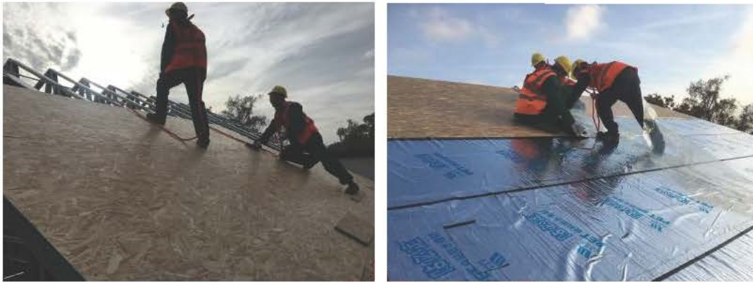
The installation of the OSB board and waterproof material for the roof.
