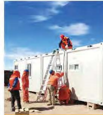
Transporting and installing
