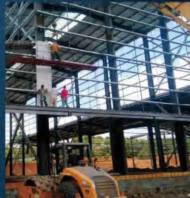
High speed of construction
