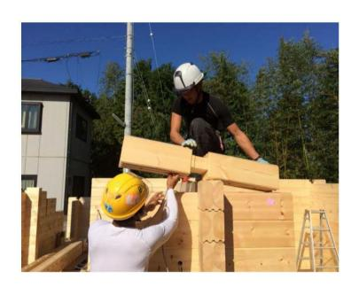
Our interlocking design increases the overall strength and durability of our log cabins. It also provides a weather tight seal. No leakage! Every log is kilndried and treated with stain on the outside and polyurethane on the inside. We also put insulation strips on every course to provide a weather tight seal.
