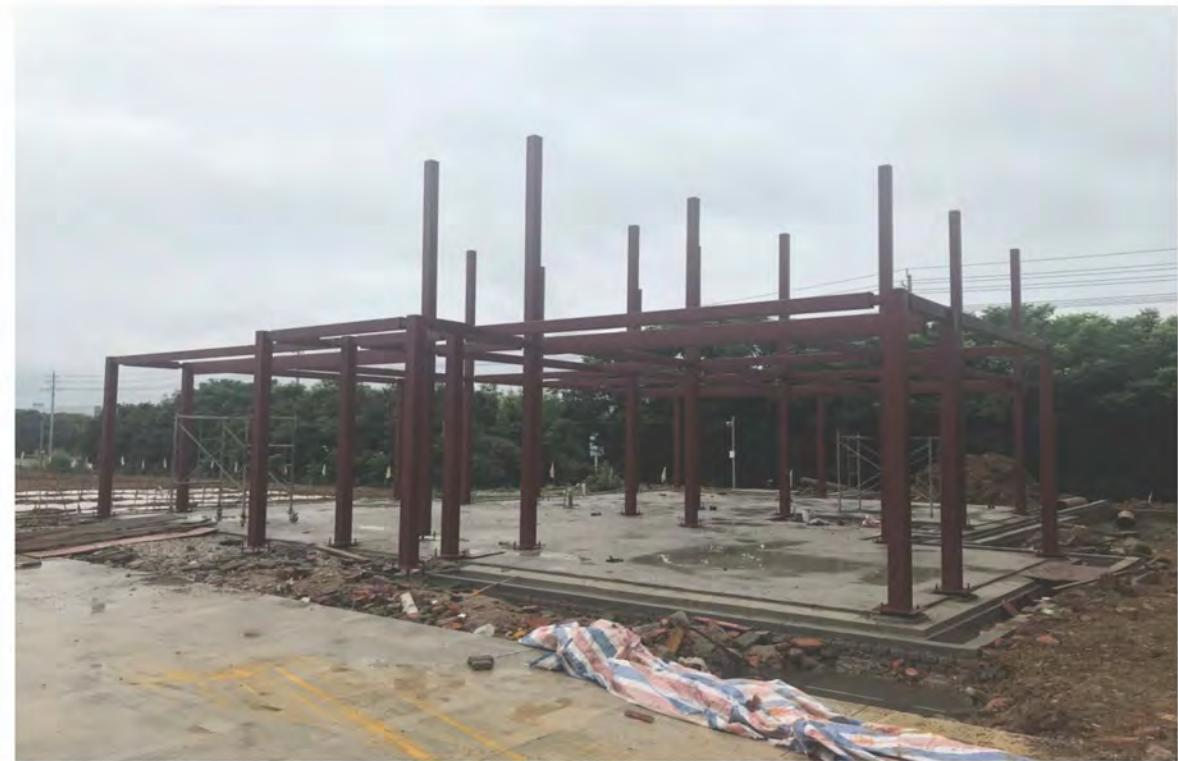
steel column and steel beam forming framework system, the use of high strength bolt connection
