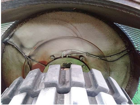
Grease top up line (TOP)
