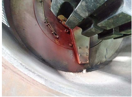
Grease top up & disposal line (BOTTOM)
