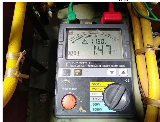
Phase W insulation resistance: 1.47 giga ohm
