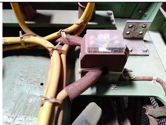
Phase U insulation resistance: 8.7 mega ohm
