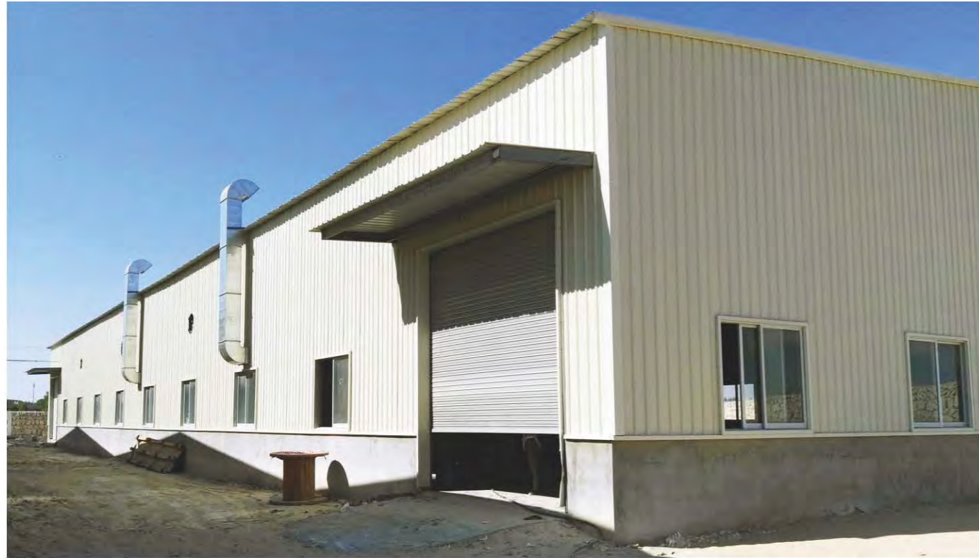
Qatar warehouse house
