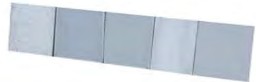
Gypsum board ceiling
