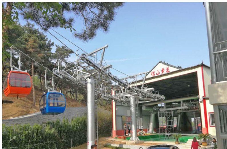
6p Cabin, Laiwu, Shandong
