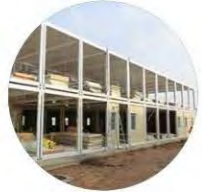
2. Install wall panels
