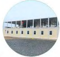
3. Install windows and door
