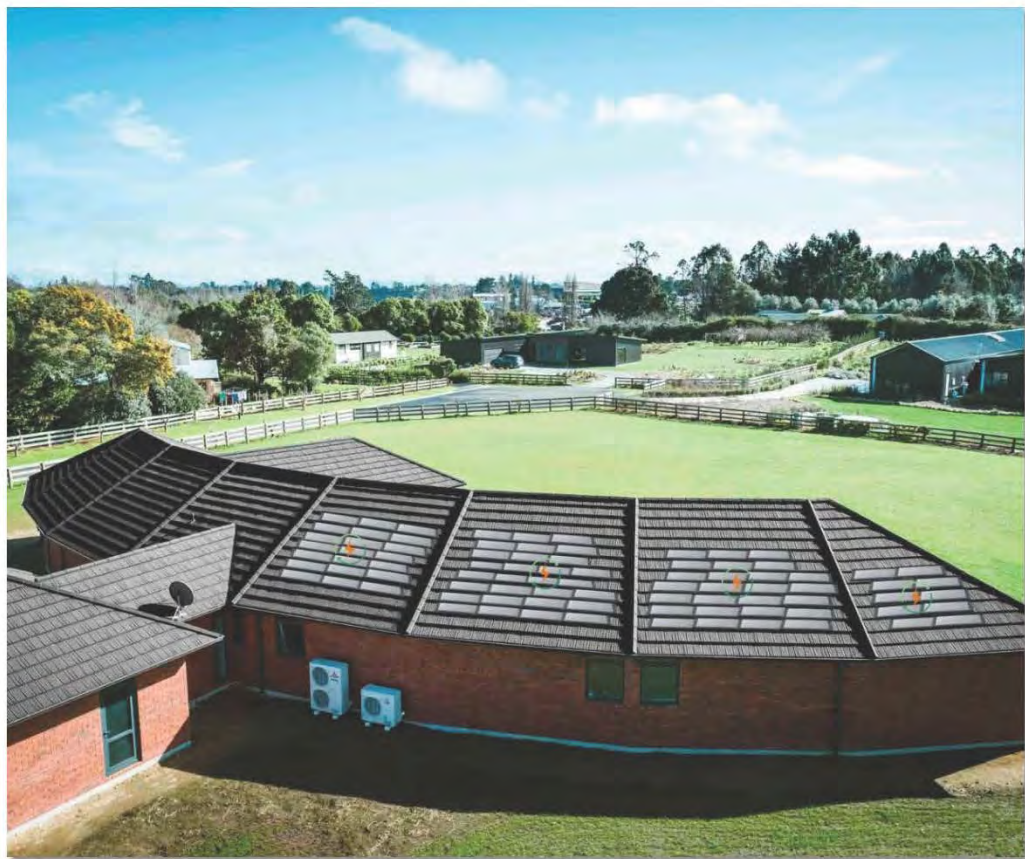
3KW SYSTEM 12KWH Power Generate Per day
