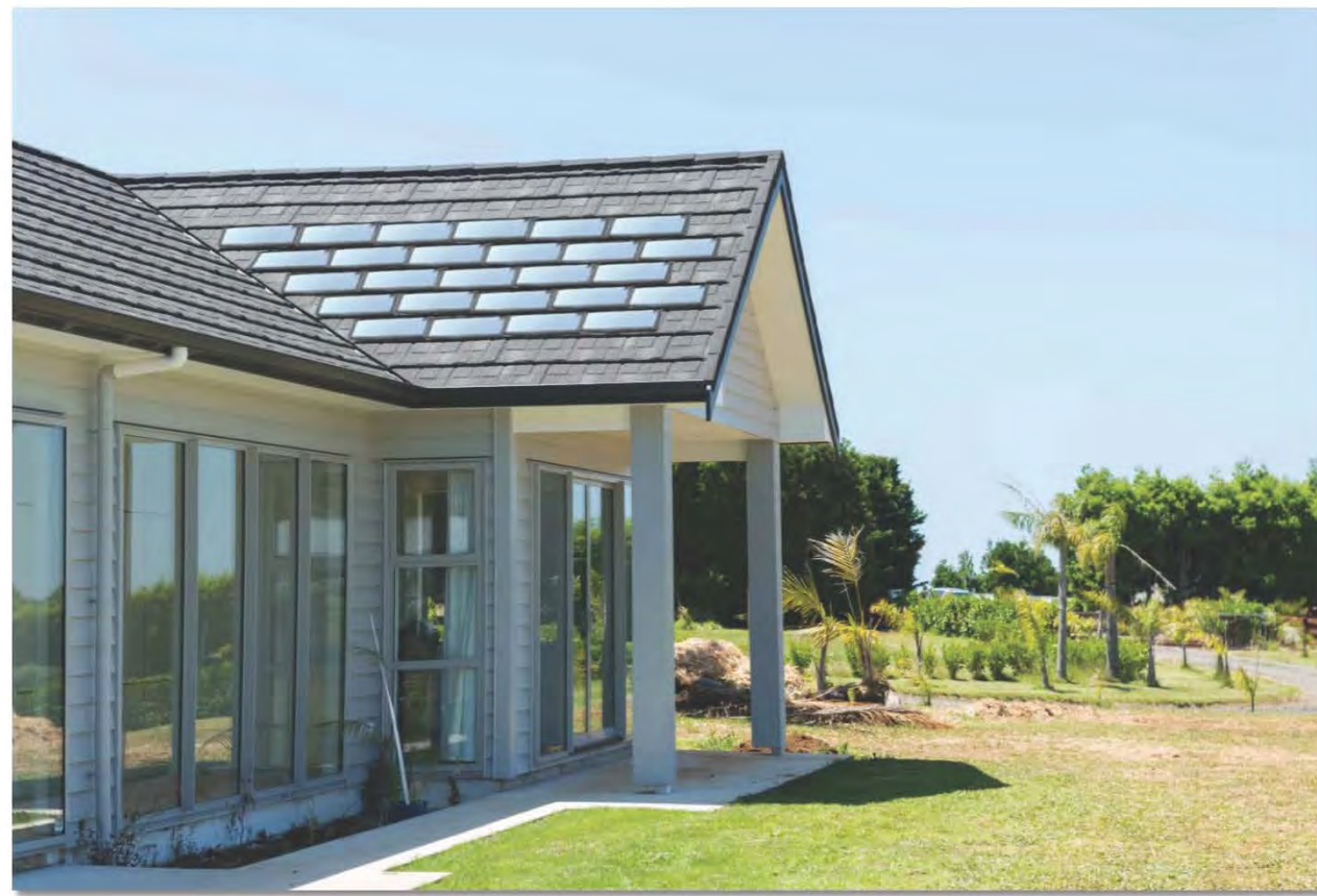
5KW SYSTEM 20KWH Power Generate Per day
