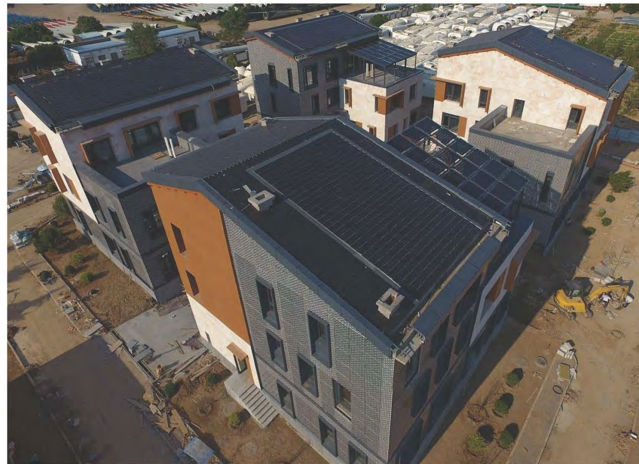
◆ Hebei Baoding Passive Residential Demonstration Light Volt Tile Roof Project (100kw)
