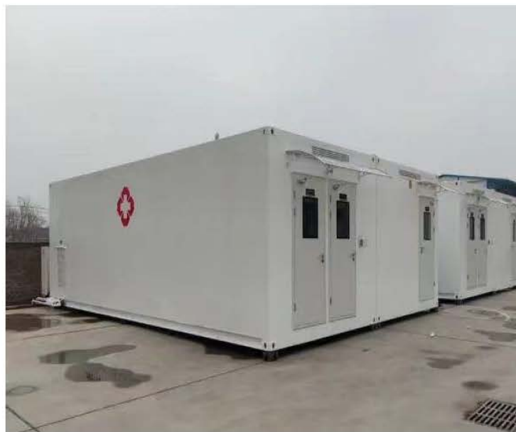
Mobile cabin hospital arranged on the field
