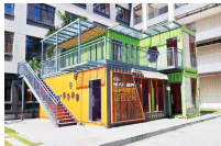
public utilities container
