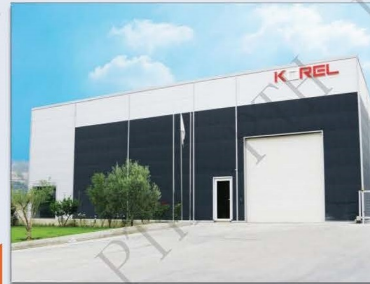
Steel structure building
