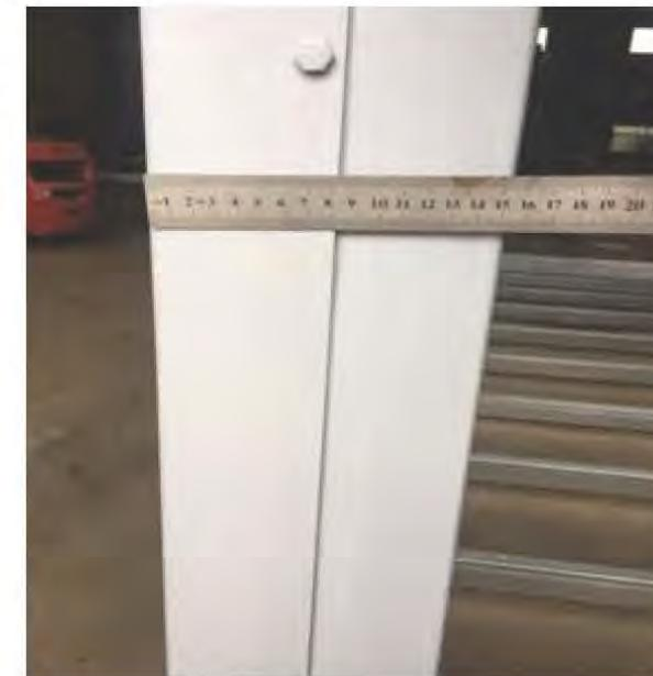
The height of the base is 27 cm, the width of the top beam is 17 cm, and the width of the column is 15 cm
