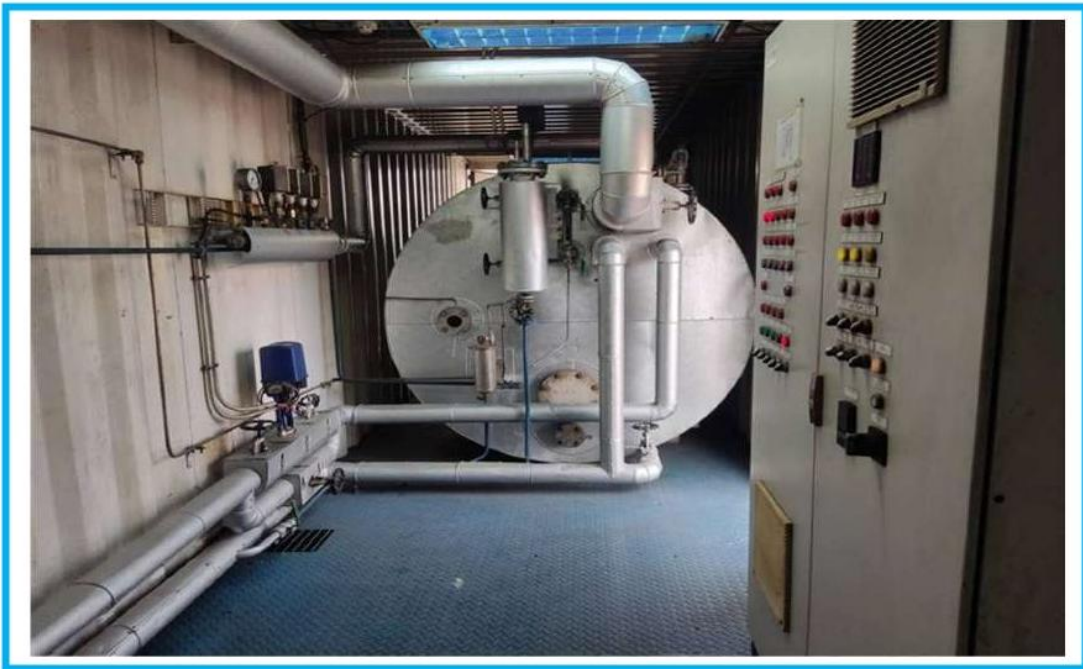
AUXILIARY BOILER
