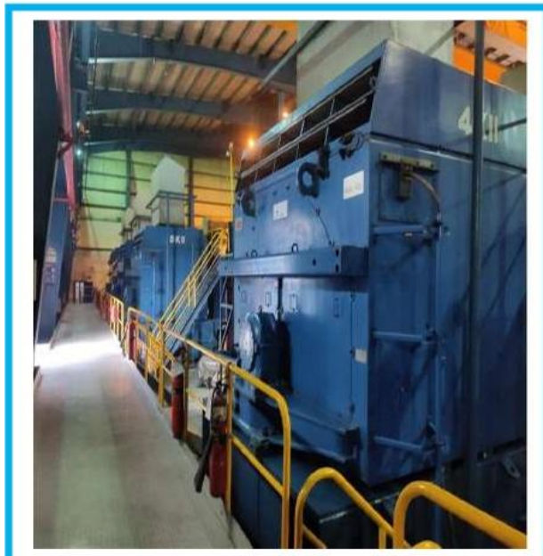
ENGINE ROOM MIDDLE FLOOR
