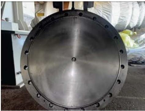
The lower outer manhole
