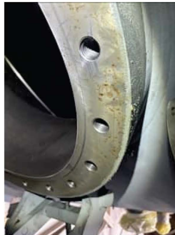
The lower outer manhole (3)
