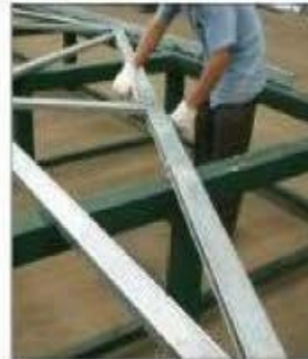
Fix the roof bolt
