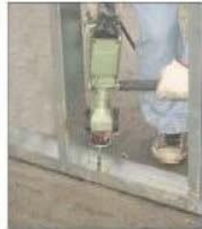
Fix expansion bolt
