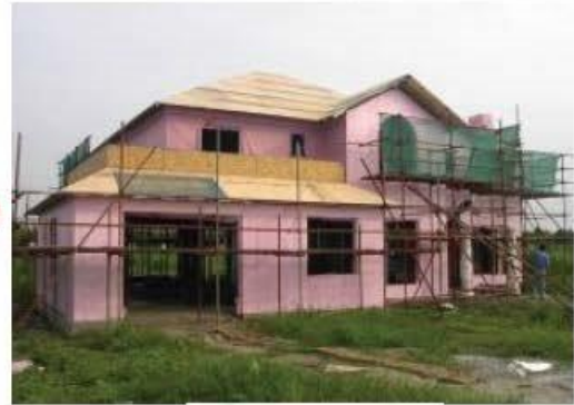
Insulation & waterproof installation
