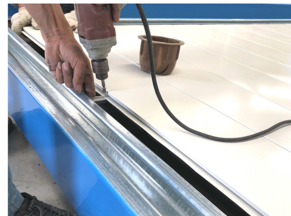
Ceiling fixing.
