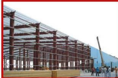
Steel structure warehouse/building
