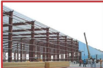
Steel structure warehouse/building
