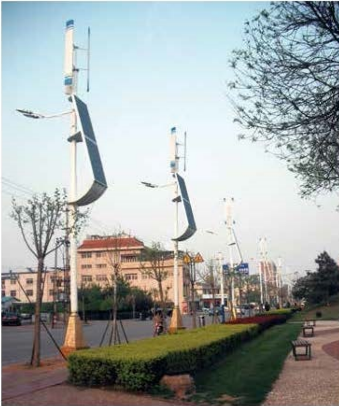
Wind & solar hybrid power supply lighting system on street
