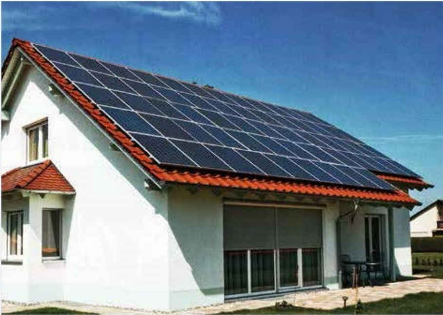
Small micro-grid power supply system in Binhai New District
