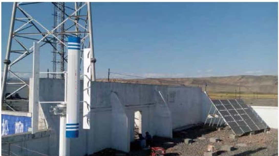
Wind & solar hybrid power supply equipment for mobile communication base station
