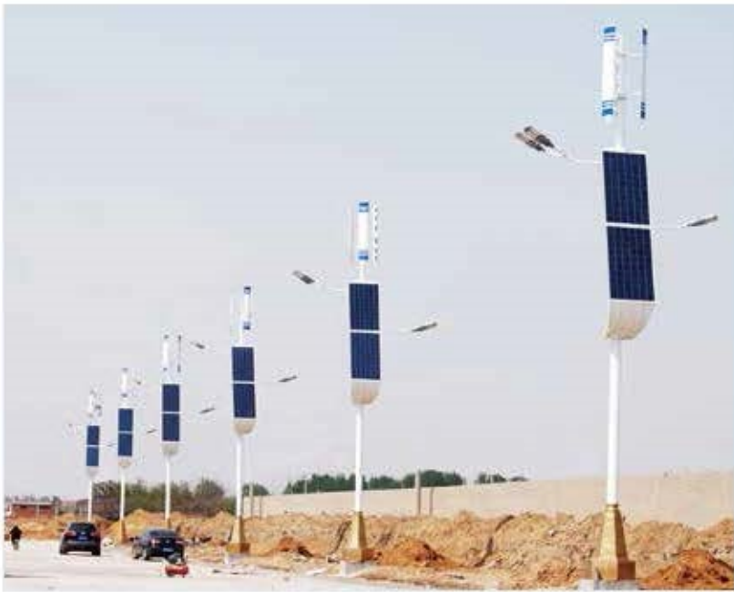
Wind & solar hybrid power supply lighting system installed in Construction site
