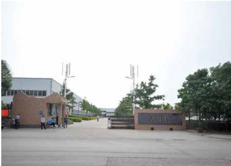
Wind & solar hybrid power supply lighting system installed in industrial zone
