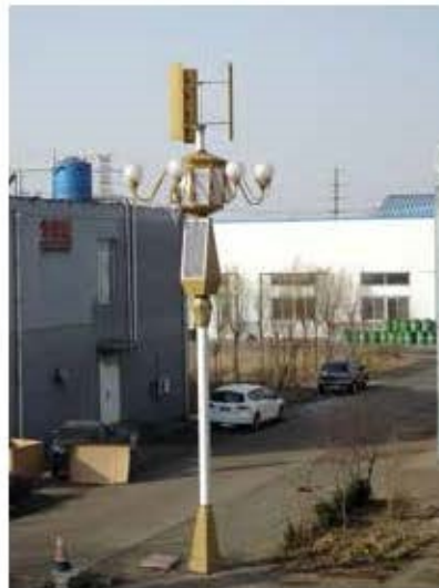
Wind & solar hybrid Chinese Style street light installed in Haigang industrial zone
