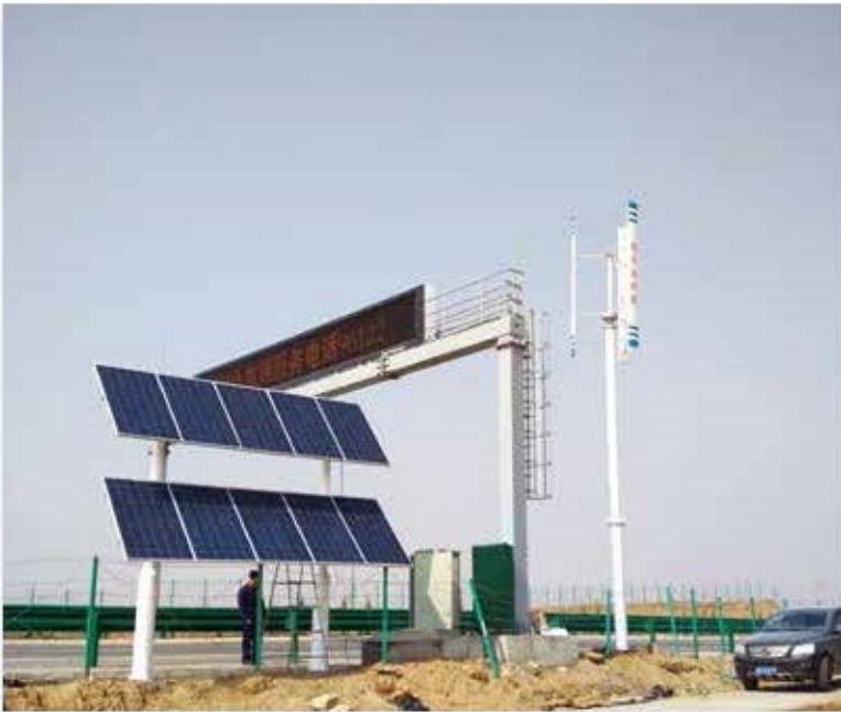
The wind solar hybrid system equipment in high speed way of Qinhuangdao
