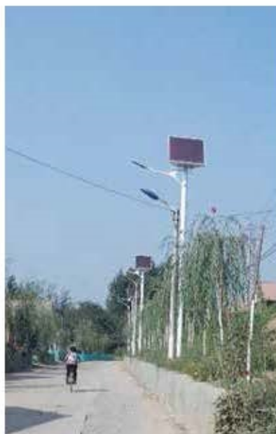
Solar street lamp at Town Fengrun
