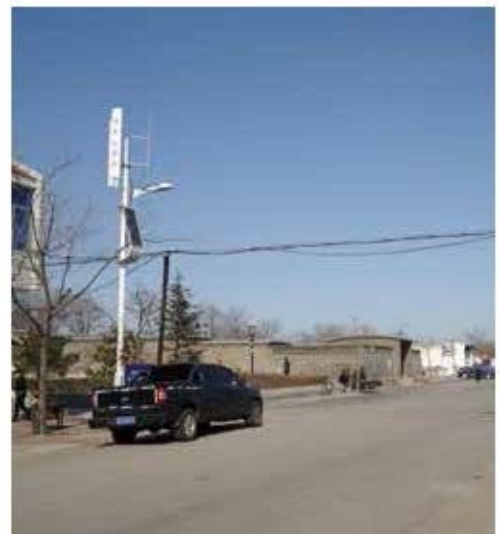
Wind & solar hybrid power supply lighting system installed in Dazhao Li Memorial Hall
