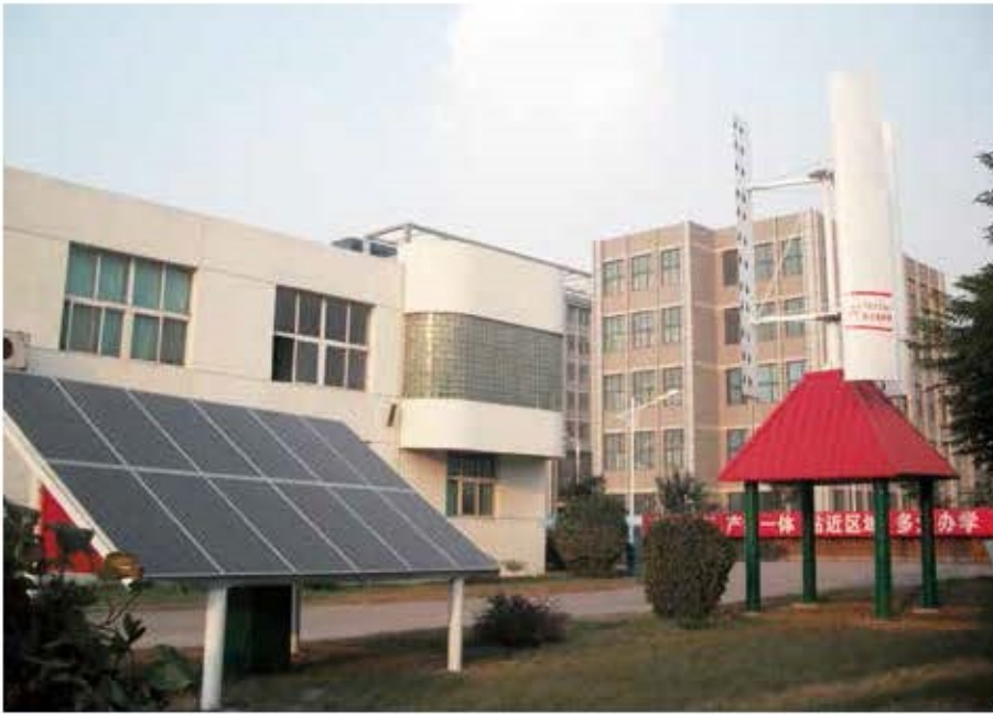
Wind & solar hybrid power supply system experimental platform in Hebei College of Industry and Technology
