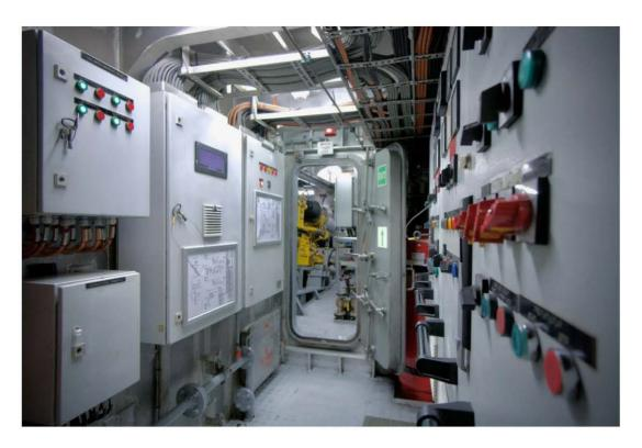
This tank room/control room is seperated from the engine room by means of watertight door.
