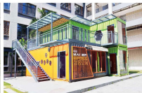
public utilities container
