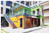
public utilities container
