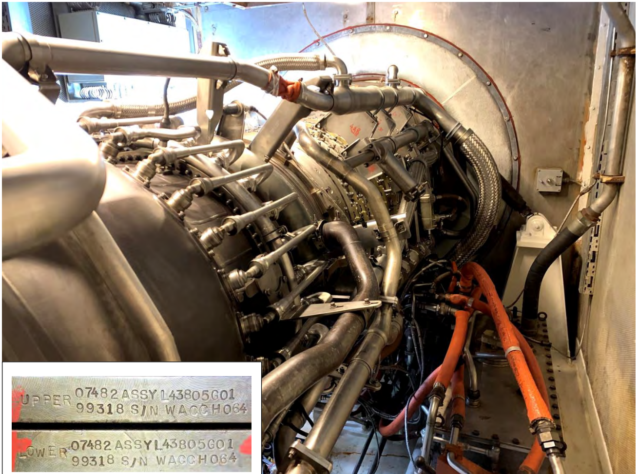
GG After maintenance
