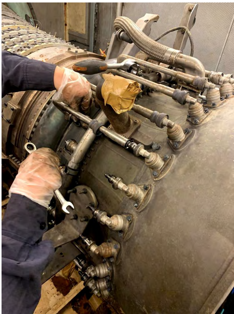
Fuel nozzle clean and Serial Number
