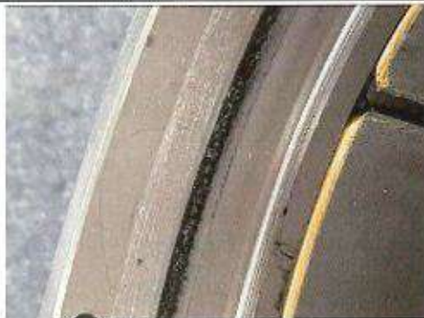
LOWER CARRIER – PITTING IN SEAL GROOVE
